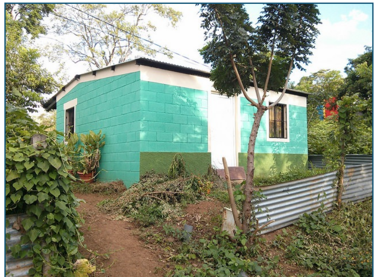
A home built by the Homes of Hope program in Nicaragua
